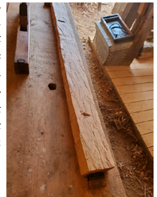
Planing is the final step for squaring the board
