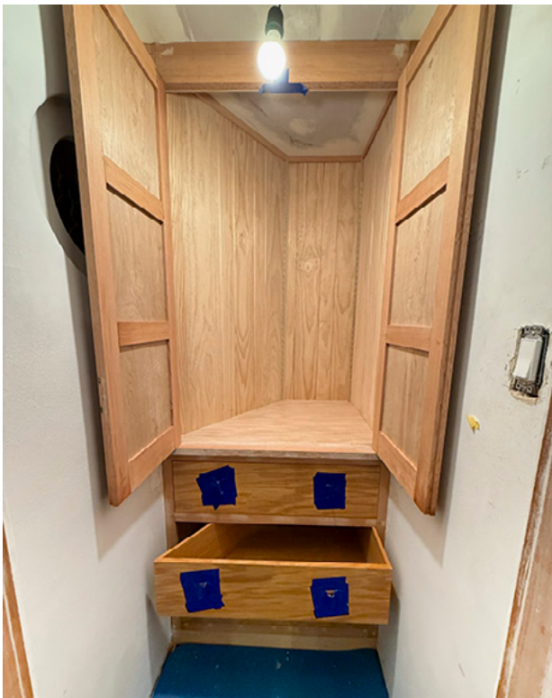
Trey and Carolyn showed a built-in cabinet they designed and built in a wedge-shaped area of their house. They used reclaimed 100-year-old Douglas fir and oak plywood for the drawer boxes. To keep the drawers aligned as they were pulled out, they used undermounted wooden runners
