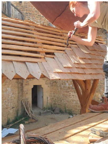
This is not a miniature, it’s just a section of the roof. Here Brittany is attaching shingles to the roof.
