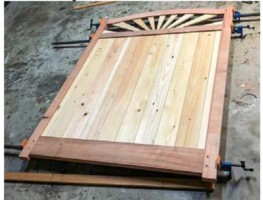
Then I assembled the frame, slid in the panel pieces, and glued the last rail in place. Again, wanting that mechanical lock, I used 1/4" dowel to drawbore the tenons, using just a 1/16" offset. Because the concrete wall leans out a little bit, I cut a small taper on the latch side of the finished gate to provide clearance and reduce the gap. Finally, Ed Sheanin came to help me hang the gate, break for lunch, and install the latch. And now it works perfectly!
