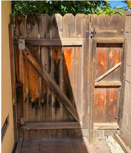
The first thing was to get rid of the old mess. Pulling it all out revealed lag screws holding the posts into either wall. Opening it all up allowed me to get accurate measurements, especially for the old lag screw holes – I wanted to avoid drilling too many new ones. Also, I wanted the new gate to span the entire width of the walkway.
