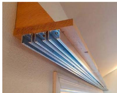
I had to check the level as I went and shim-out a few of the triangular braces up above to maintain the proper angle all the way along.
