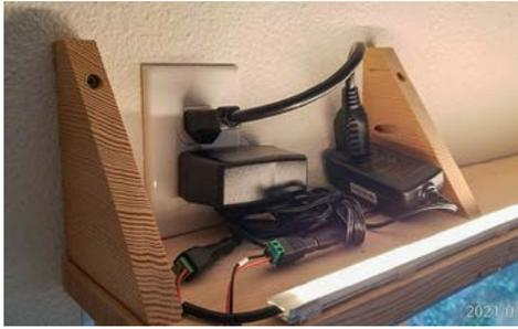
The LED strips each require 12 volts DC at 2.5 amps. I had bad luck with a 6-amp power supply so I ended up just using two 3-amp supplies. (In hindsight, I wish I had run low-voltage wiring all the way down to the switchbox, which would have enabled me to set up dimmer controls for both LED strips. But with the 120V line feeding the power supplies up top, I cannot put dimmers ahead of those power supplies.)
