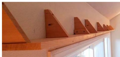
Here you see the installed header board and the braces. These are screwed into wall studs for structural support.
